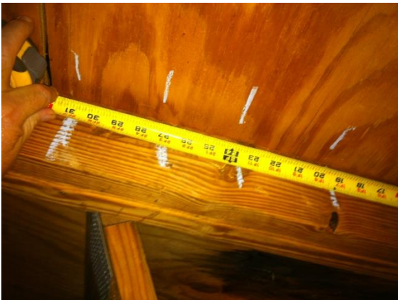
SHEATHING NAIL SPACING
