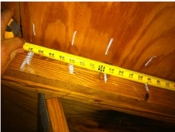
SHEATHING NAIL SPACING
