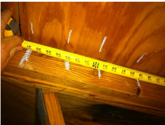
SHEATHING NAIL SPACING
