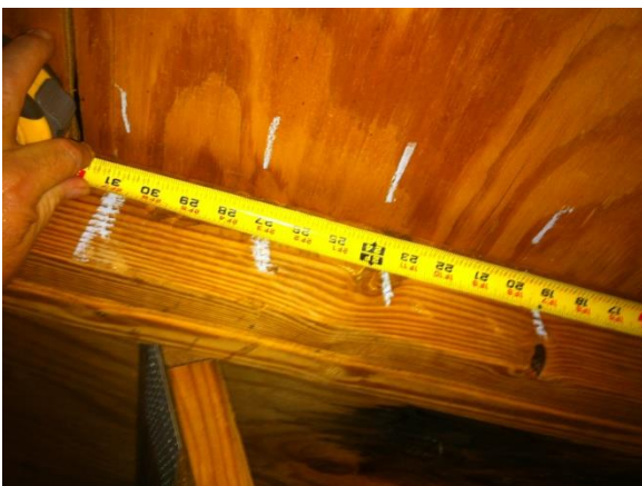
SHEATHING NAIL SPACING
